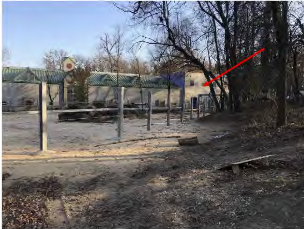
Photo #9. View of Valley Habitat and Elephant barn. Red arrow indicates location of the new 50 foot addition to the barn.
