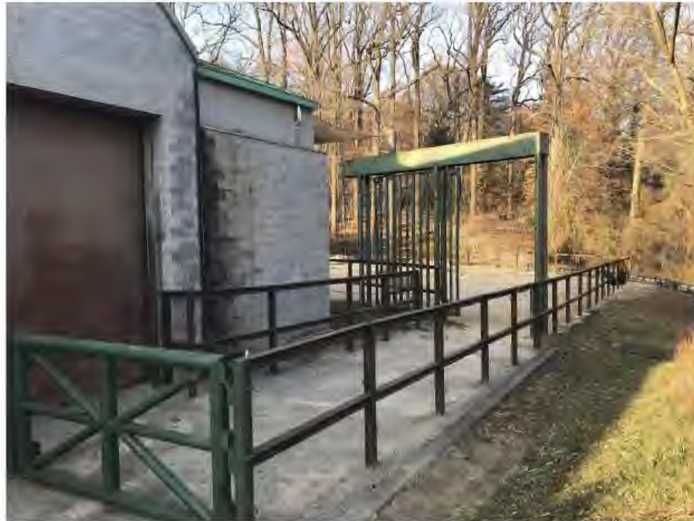
Photo #12. View of the Forest Yard. Brown roll up door on the left is the animal door into the chute into the exhibit. Green gate is the shift gate from the chute into the Forest Yard. Note: this area will be renovated in spring of 2019 as part of the overall renovation of the elephant barn and exhibits.
